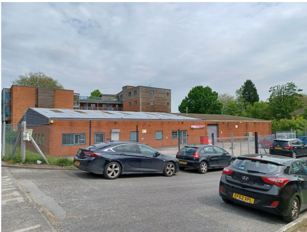
Application site together with single storey building to be demolished and Quadrangle residential apartment in the background, the access road into Albany Road Trading Estate is in the foreground
