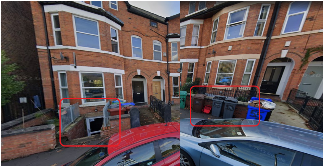
Door to basement of number 51 Albany Road (to the left) and basement window to 55 Albany Road as referenced in the assessment
